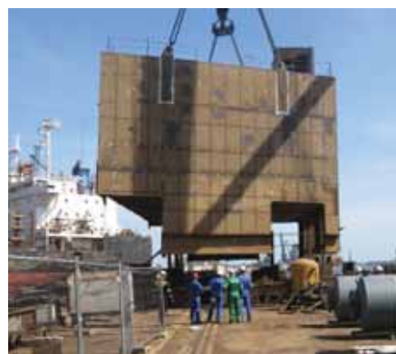
Engine room being lowered onto the deck of the Freja Pacific.
